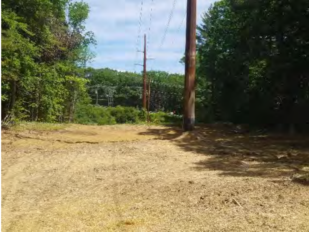
Fig 5: Str. 33 work area restored. Viewing north. (06-08-20).
