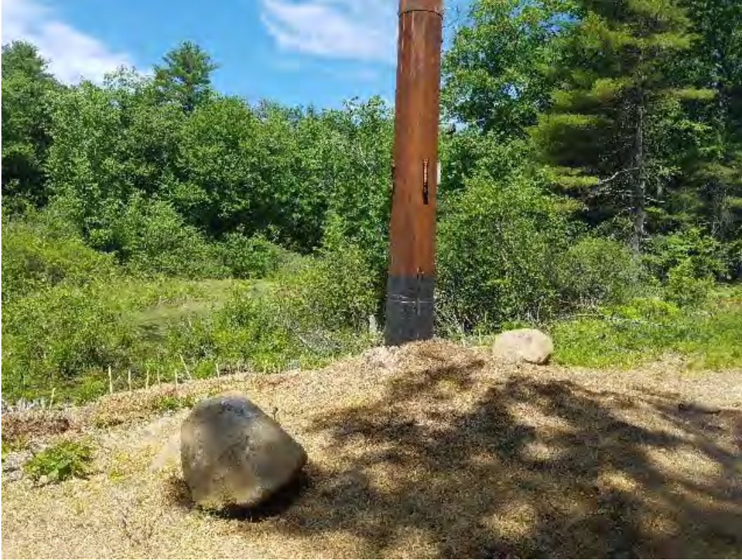
Fig 7: Str. 34 work area restored. Viewing northwest. (06-08-20).
