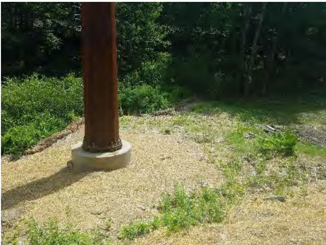
Fig 14: Str.28 and wetland DW49 restored. Viewing east. (06-10-20).
