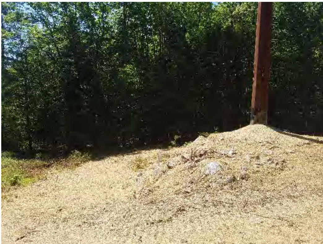
Fig 2: Str. 74 work area restored. Viewing south. (06-04-20).
