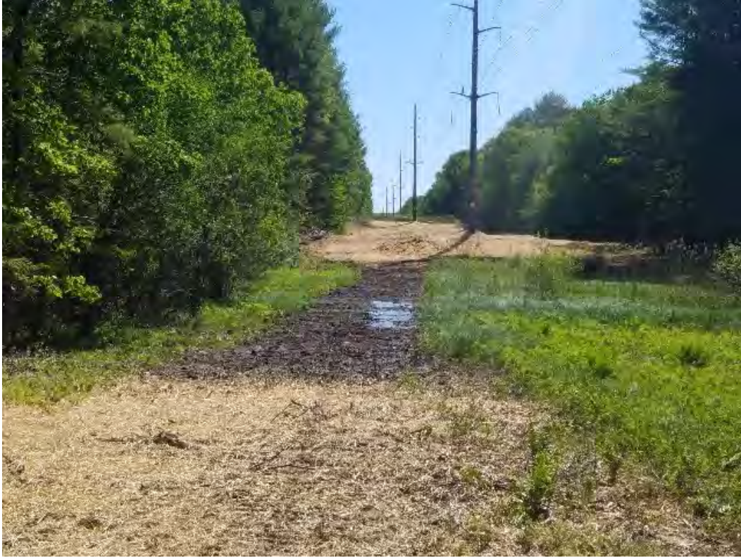
Fig 3: Access road between Strs. 74-75, through wetland DW21, restored. Viewing east. (06-04-20).
