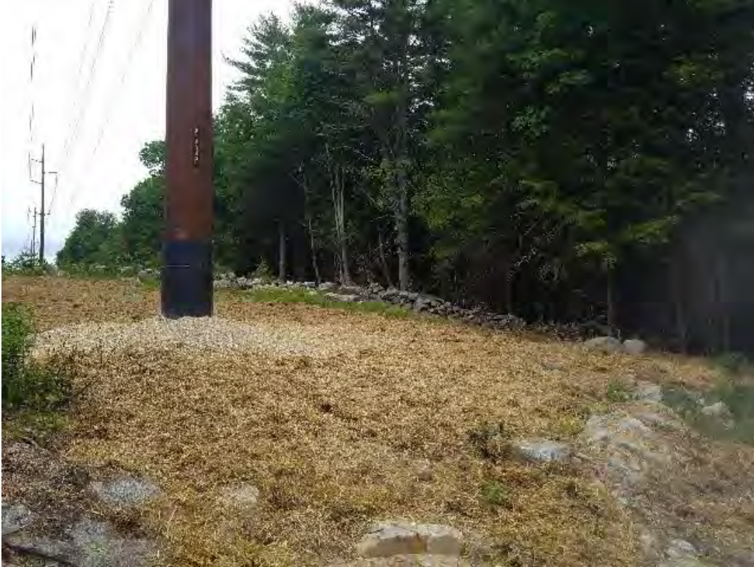
Fig 11: Str. 83 work area restored. Viewing northwest. (06-09-20).
