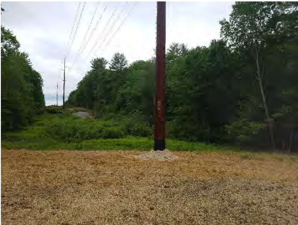
Fig 12: Str. 82 work area restored. Viewing east. (06-09-20).
