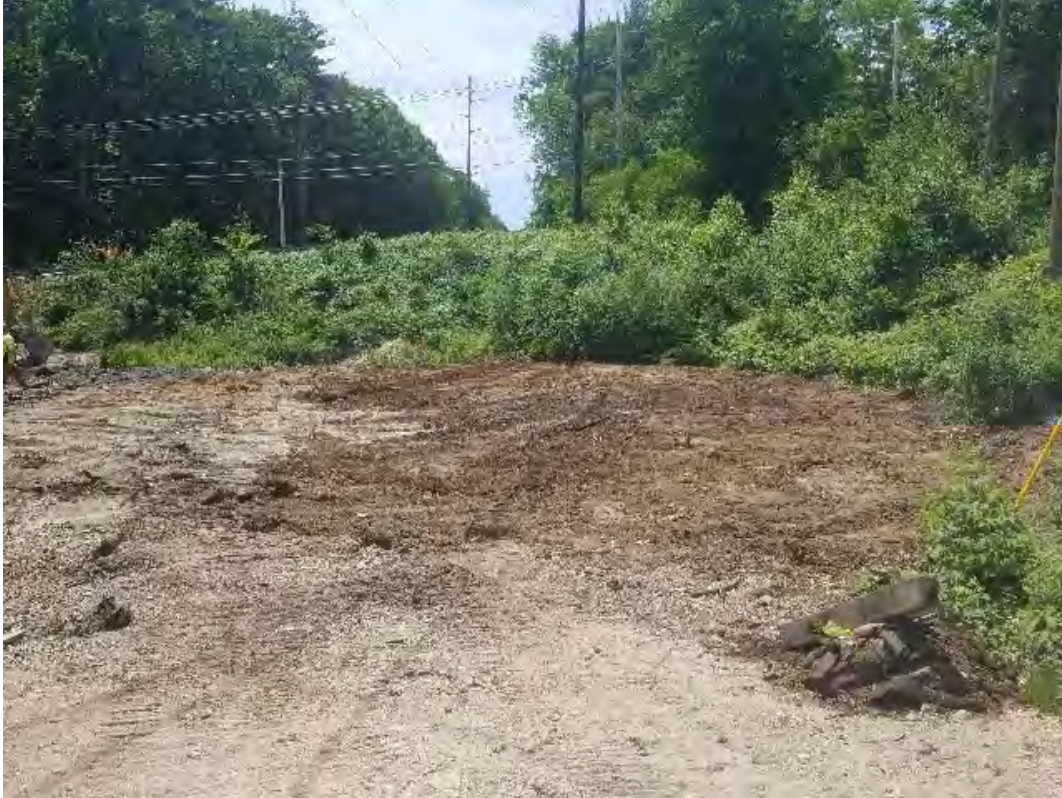
Fig 15: Restored dewatering basin area at Str. 32. Viewing south. (06-10-20).
