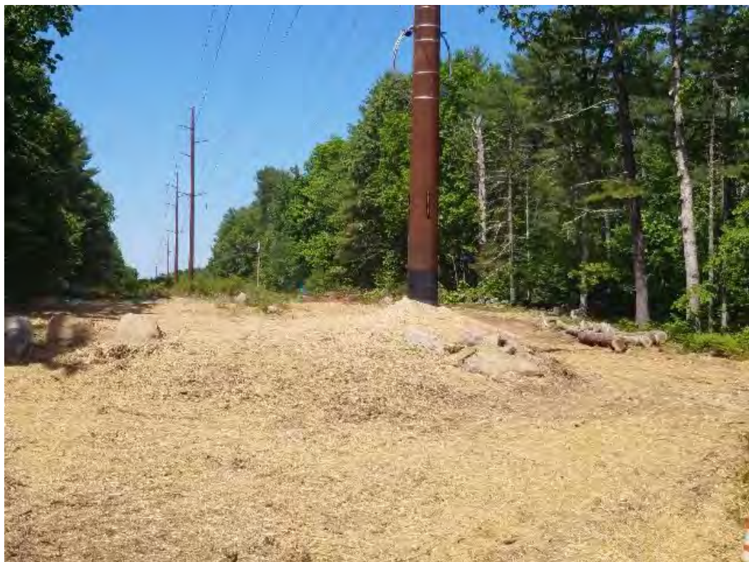
Fig 4: Str. 67 work area restored. Viewing west. (06-04-20).
