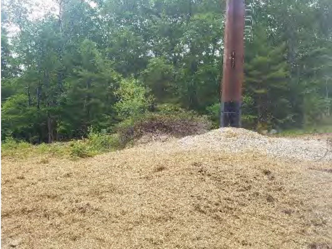
Fig 9: Str. 84 work area restored. Viewing southeast. (06-09-20).
