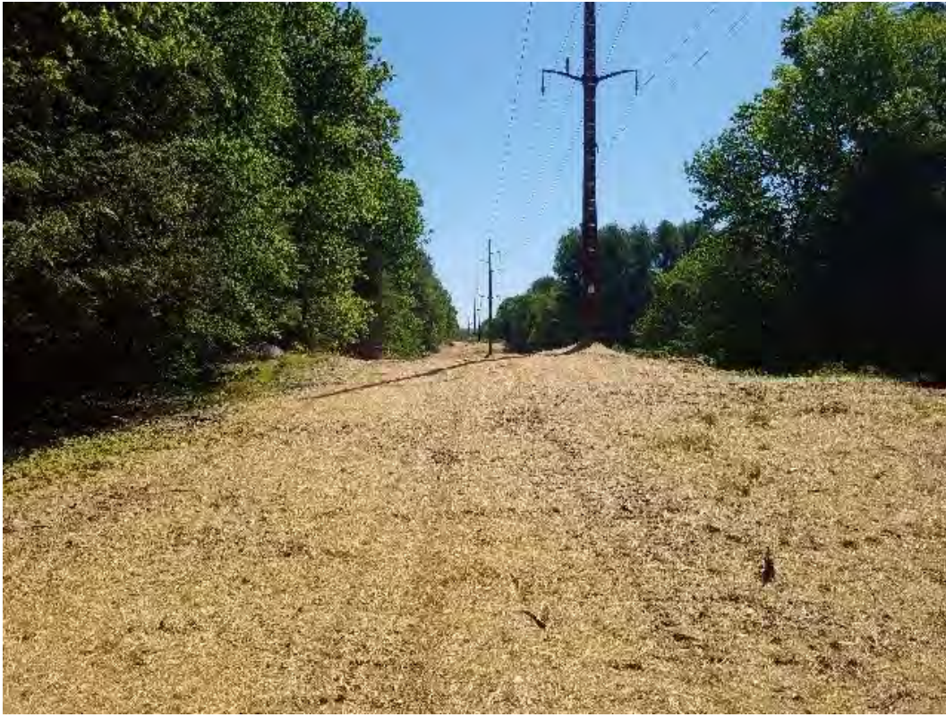
Fig 1: Str. 73 work area restored. Viewing east. (06-04-20).
